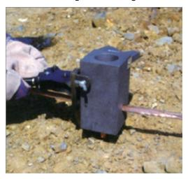
**Step-05:** Close the clamp tightly once the conductors are properly positioned.
