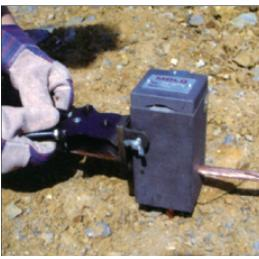
Step-07: Next, take a bag of properly sized welding material (as identified on the mold ID tag) out of the box. Remove the lid over the mold crucible. Quickly pour the loose welding material powder into the mold. Pour 1/4 to 1/3 of the starting material over the welding material in the mold crucible. Close the lid and pour the remaining 3/4 to 2/3 of the starting material into the slot on the mold cover.
