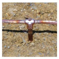
Open the mold and remove the connection. Use care to prevent chipping the mold. Avoid contact with hot materials. Completed EXOTHERMIC WELDING connection.
